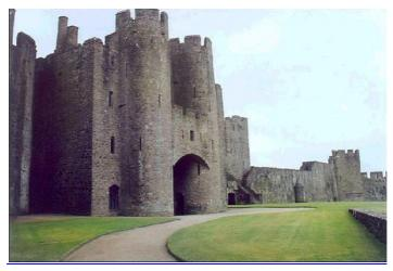
Source: Pembroke Castle with its integrated gatehouse and expanded neck built from ca. 1093.<sup>61</sup> Notice that the towers are round.
